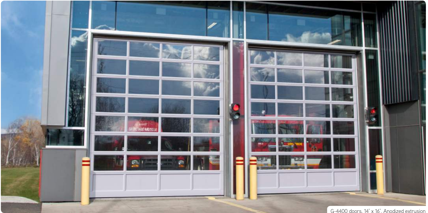
G-4400 doors, 14' x 16', Anodized extrusion
